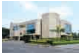
SBU Block (2nd floor), Hazira
