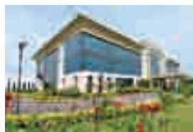
Administrative Building, Vadodara
